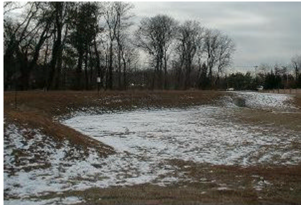
A dry extended detention pond is designed to temporarily detain runoff during storm events
