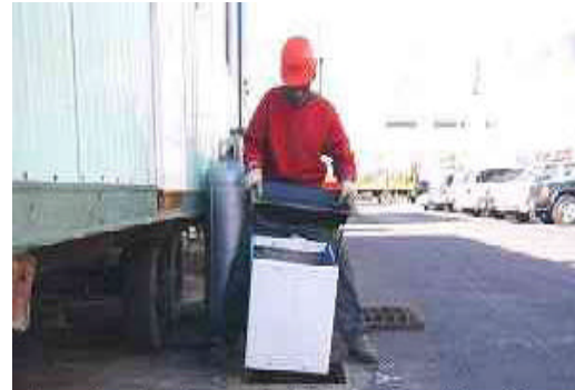
A worker inserts a catch basin insert for oil and grease, trash, debris, and sediment removal from storm water as it enters the storm drainage system (Source: AbTech Industries, 2001)
